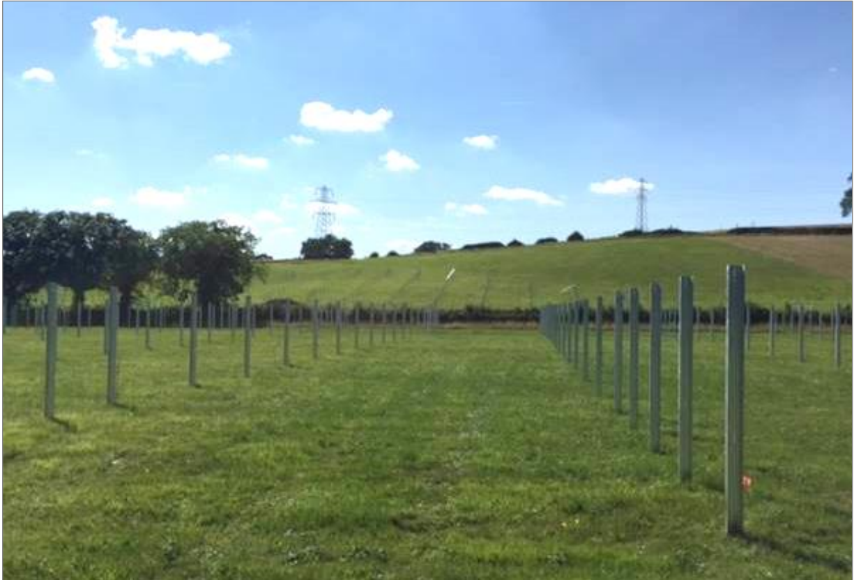
Figure 4-2: Piles for a solar farm in place (image supplied by Infinergy UK)
